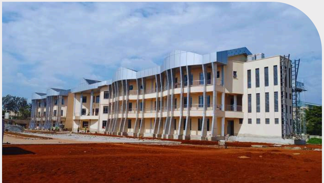
PHOTO: LVBC headquarters under construction
